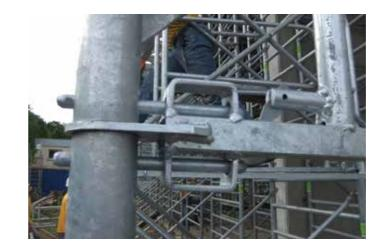
The shoring towers built by elements, once assembled, form a rigid, very safe structure.
