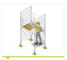
7<sup>th</sup> **STAGE**Place the platforms on the element bars.
